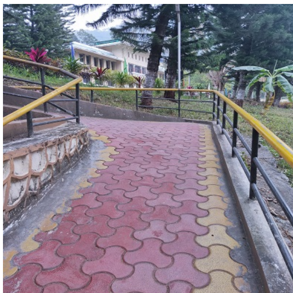
Ramps with railing
