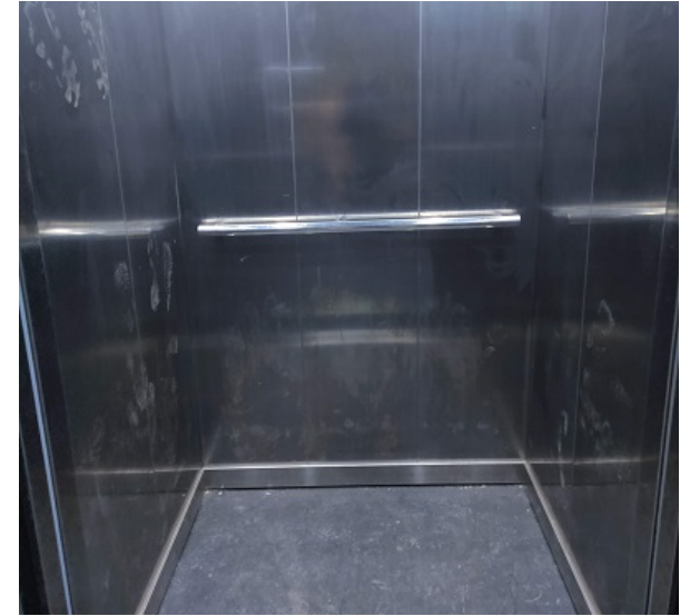
Lift Facilities at Academic Blocks
