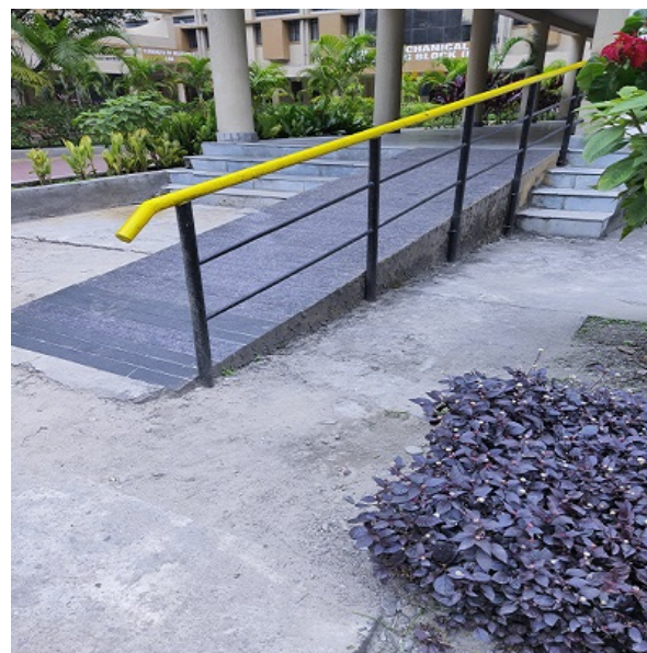
Ramps with railing
