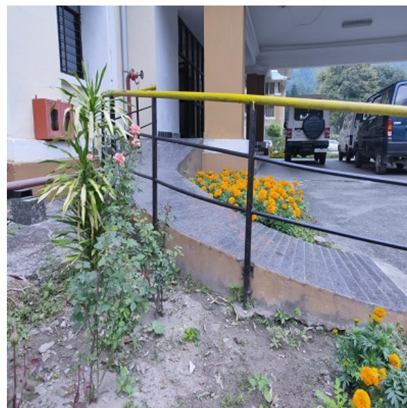
Ramps with railing
