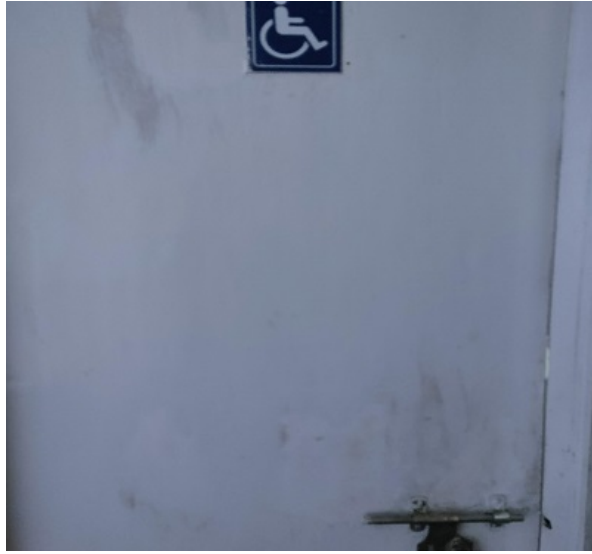
Toilets for divyangjan
