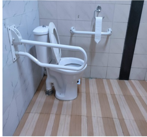
Toilets for divyangjan
